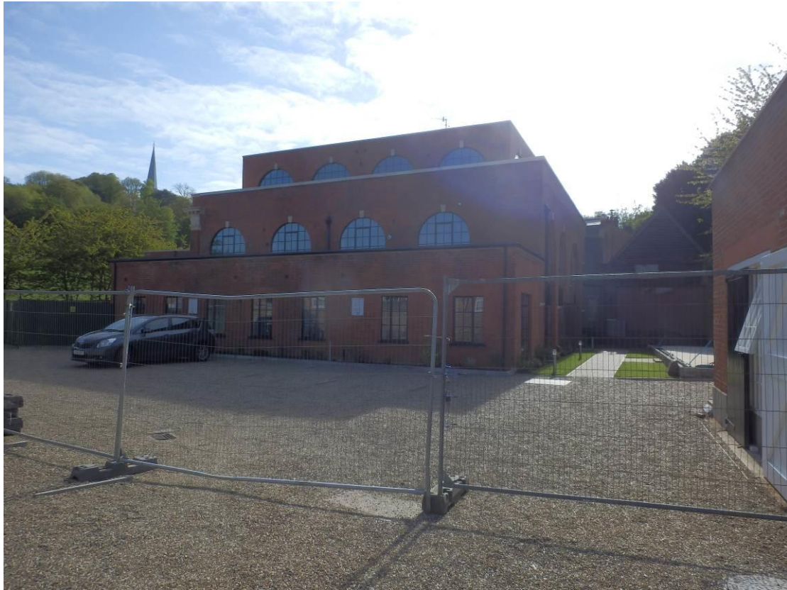
Western elevation of the property
